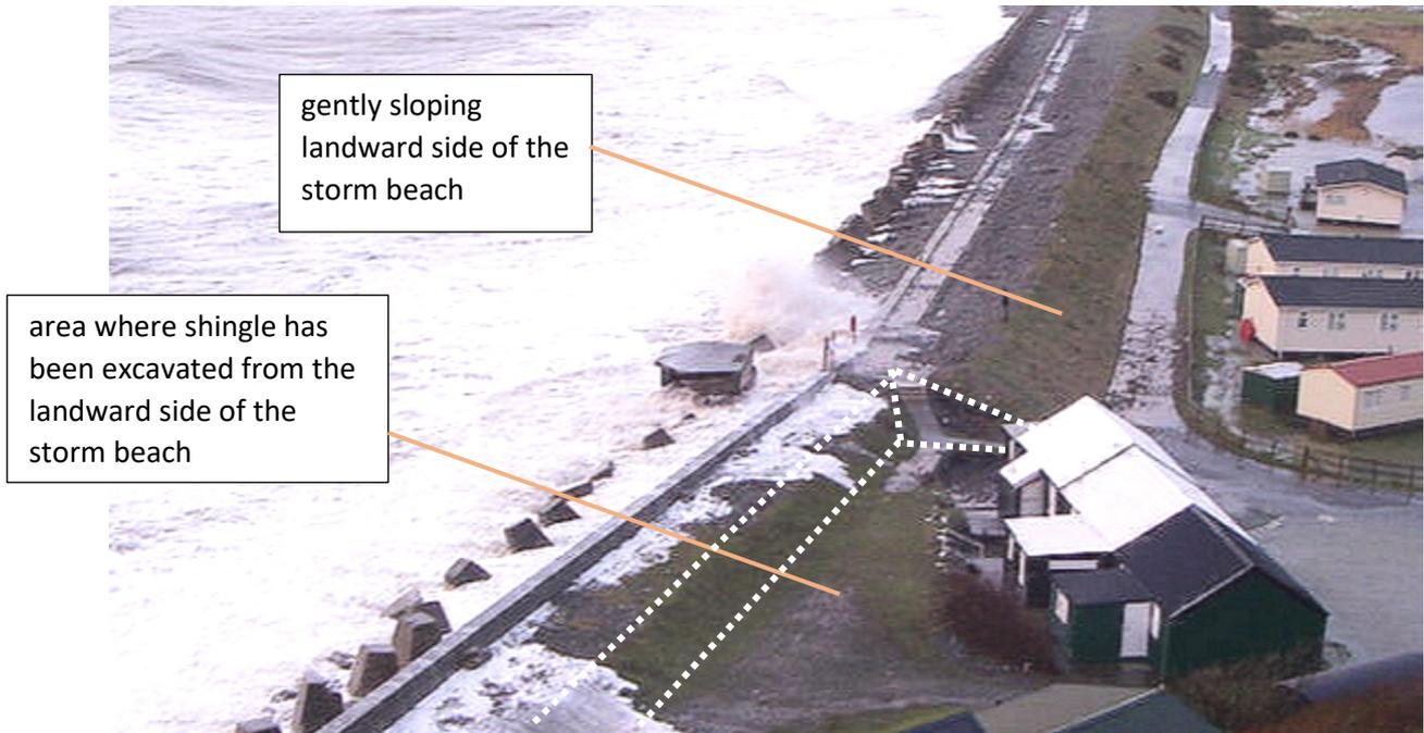
**Figure 31:** Friog corner under storm conditions, before reconstruction of the sea wall.
