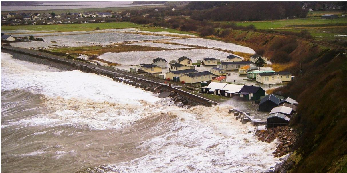
**Figure 22:** Failure of the eroded section of the Ro Wen shingle spit at Friog corner during a storm, causing localised flooding.
