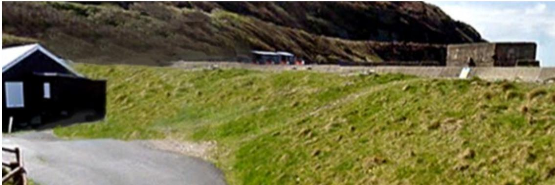
**Figure 37b:** Suggested relocation of the huts further from the sea wall, with restoration of a substantial embankment to provide support for the concrete wall.
